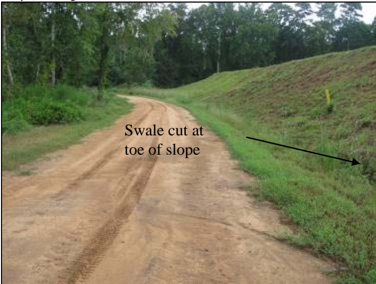
Photo 31: Ash Pond – West embankment exterior slope, toe of slope and road looking north.
