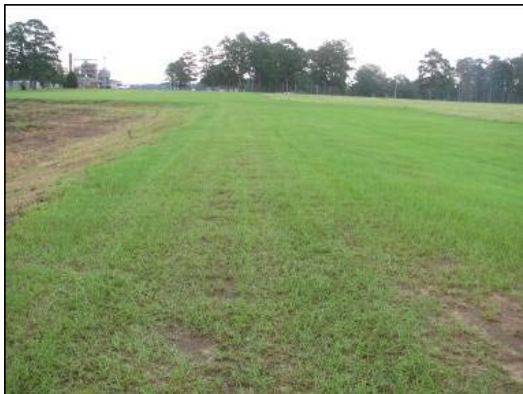
Photo 41: Ash Pond – Crest South Embankment looking east.
