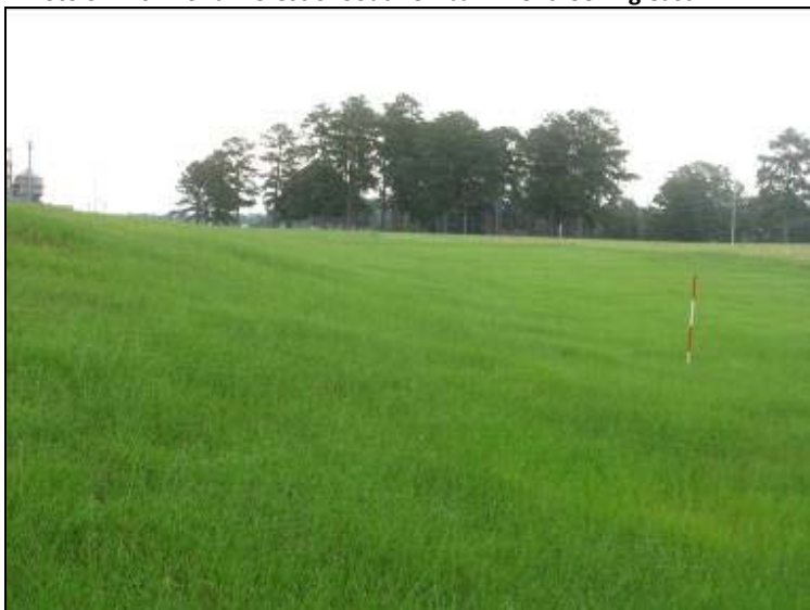
Photo 39: Ash Pond – South embankment exterior slope, looking east.
