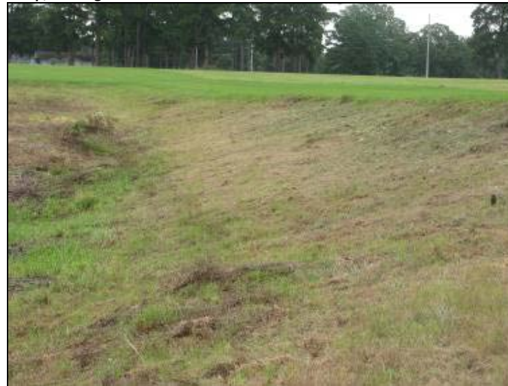
Photo 72: Ash Pond – South embankment interior slope, looking east.
