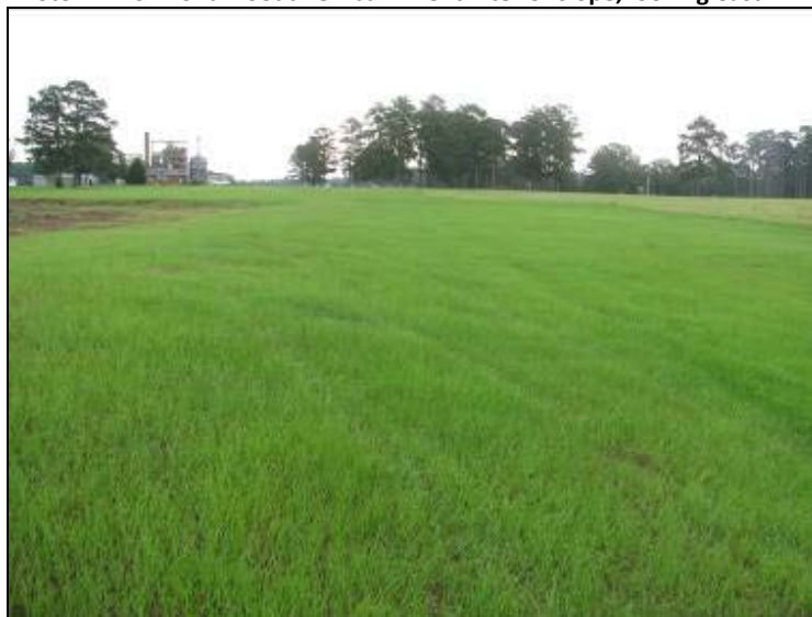
Photo 44: Ash Pond – South embankment exterior slope, looking east.
