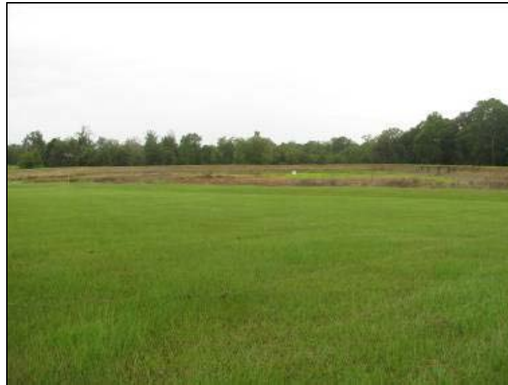
Photo 56: Ash Pond – General view of Ash pond, looking west.
