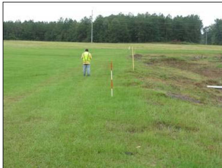
Photo 58: Ash Pond – Crest of southeast embankment near northeast corner, looking southwest.
