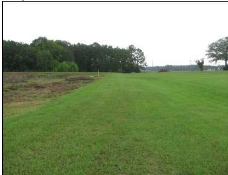
Photo 48: Ash Pond – Crest of southeast embankment near southeast corner, looking northeast.
