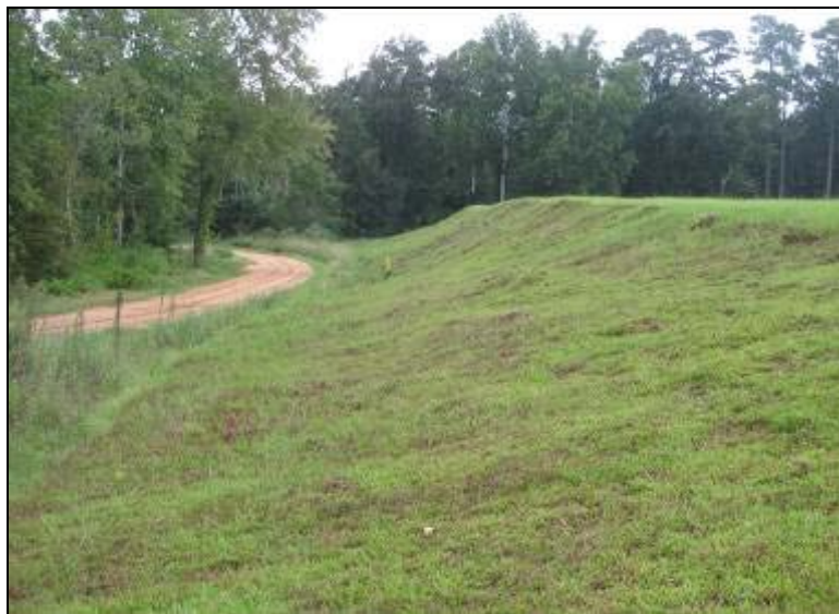
Photo 33: Ash Pond – West embankment exterior slope near southwest corner, looking north.
