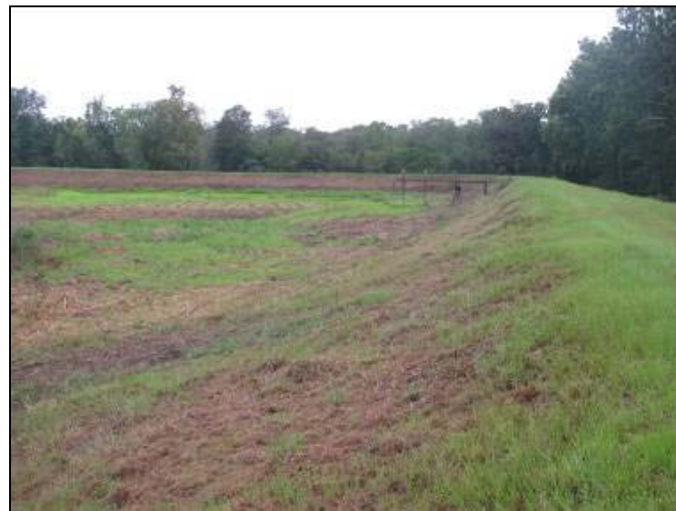
Photo 2: Ash Pond – North embankment interior slope, looking west.
