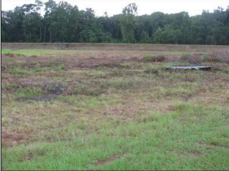
Photo 49: Ash Pond – General view of pond surface area near southeast corner, looking northwest.
