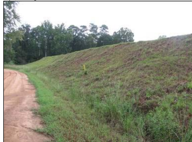
Photo 32: Ash Pond – West embankment exterior slope near southwest corner, looking north.
