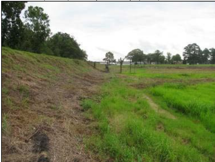
Photo 67: Ash Pond – North embankment interior slope, looking east.
