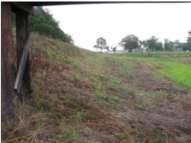
Photo 9: Ash Pond – North embankment interior slope, looking east.
