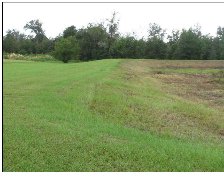
Photo 46: Ash Pond –Crest of South embankment near southeast corner looking west.
