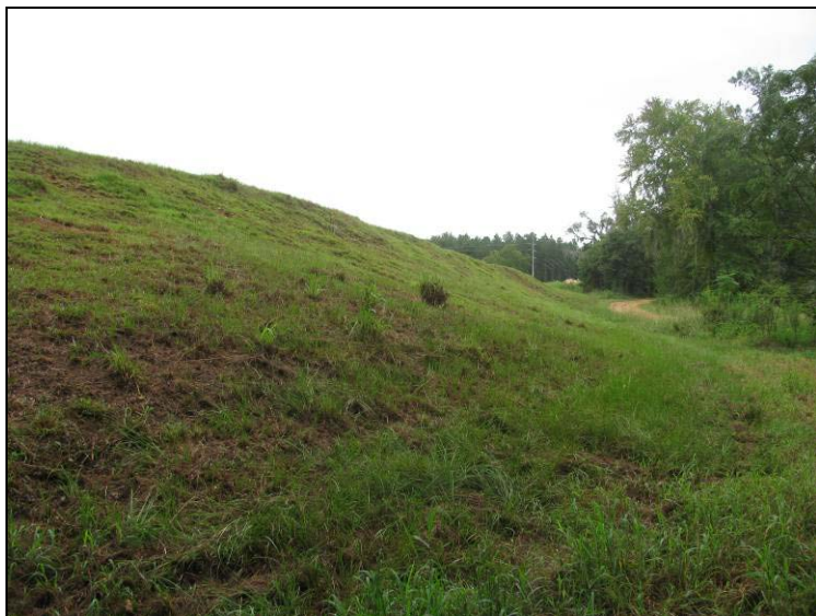
Photo 17: Ash Pond – West embankment exterior slope near northwest corner, looking west.
