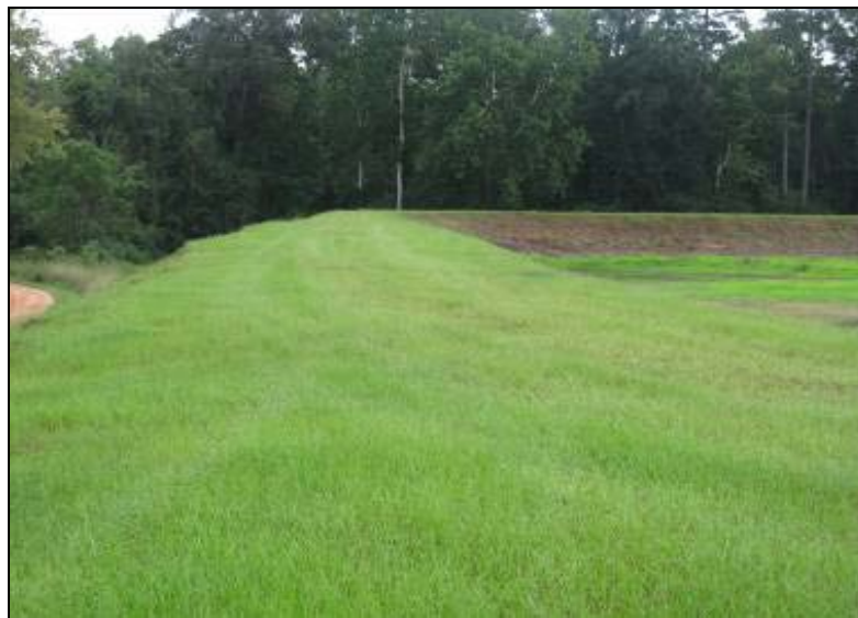
Photo 34: Ash Pond – Crest of west embankment looking north.
