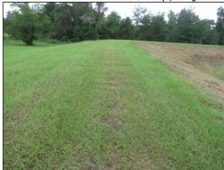
Photo 40: Ash Pond – Crest of south embankment looking west.
