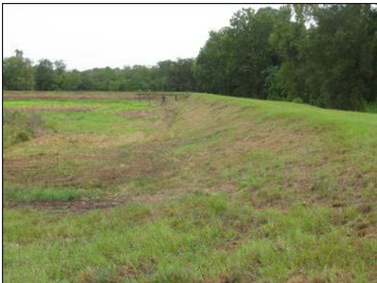
Photo 57: Ash Pond – North embankment interior slope near northeast corner, looking west.
