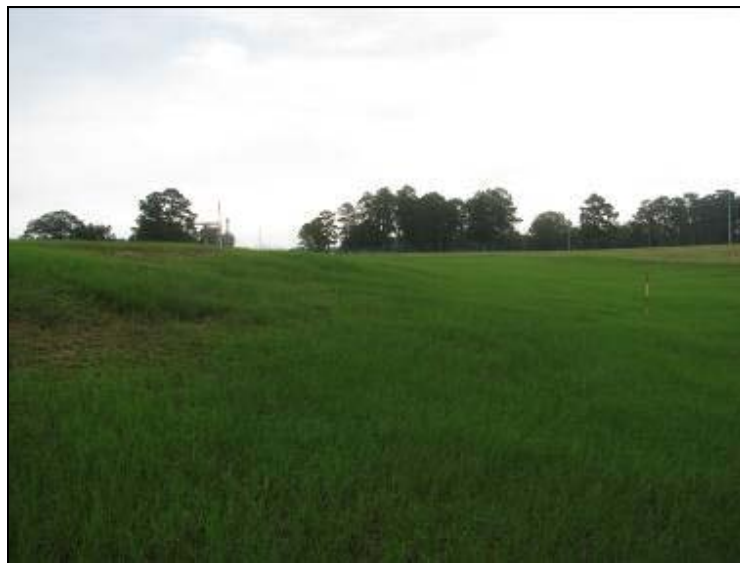
Photo 38: Ash Pond – South embankment exterior slope, looking east.
