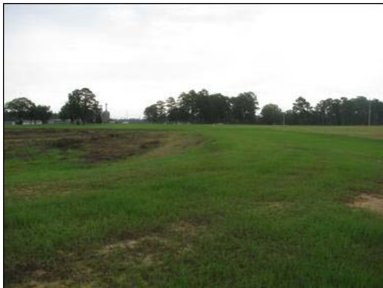
Photo 37: Ash Pond – Crest of South embankment looking east.
