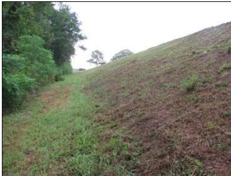
Photo 14: Ash Pond – North embankment exterior slope, looking east.
