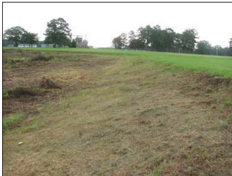
Photo 42: Ash Pond – South embankment interior slope, looking east.
