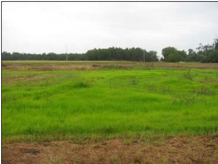
Photo 13: Ash Pond – General view of pond bottom surface, looking south.
