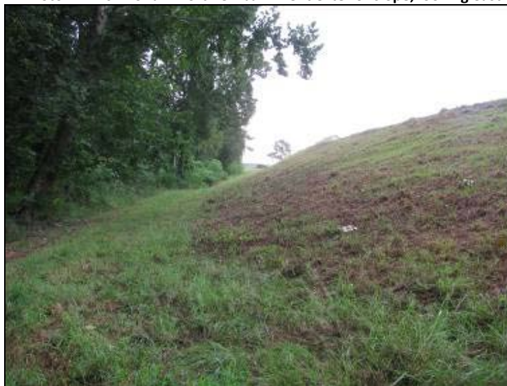
Photo 16: Ash Pond – North embankment exterior slope near northwest corner, looking east.
