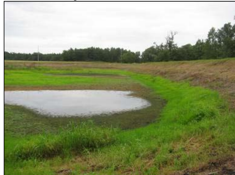
Photo 68: Ash Pond – West embankment interior slope, looking south. Note: ponded water near northwest corner of pond.
