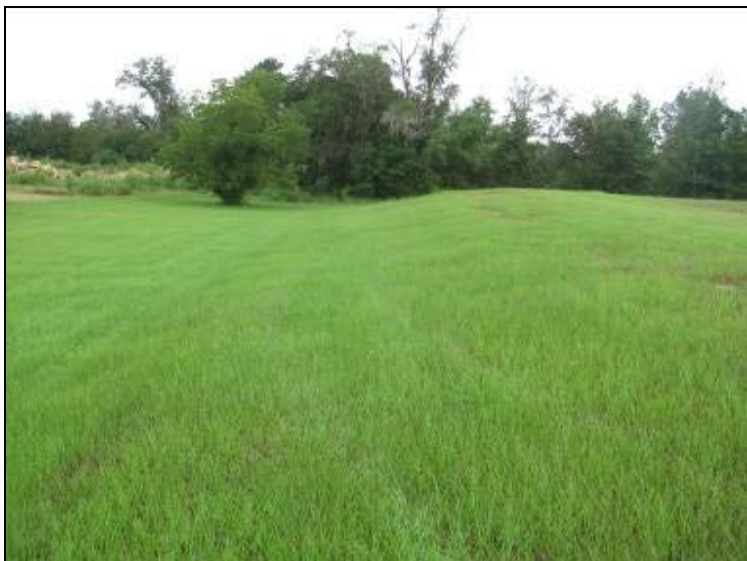
Photo 45: Ash Pond – South embankment exterior slope, looking west.
