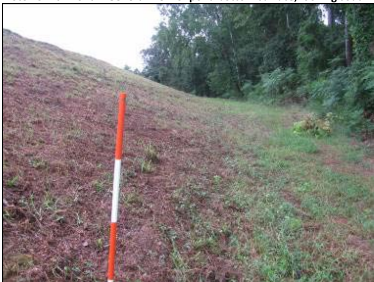
Photo 15: Ash Pond – North embankment exterior slope, looking west.
