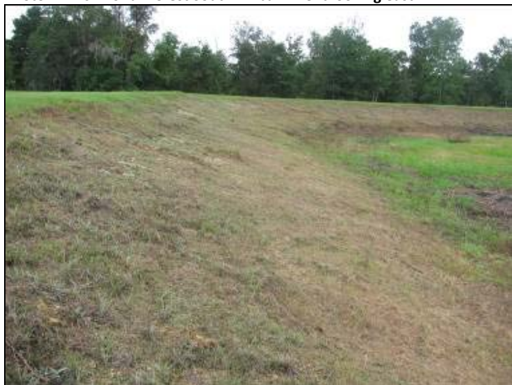
Photo 43: Ash Pond – South embankment interior slope, looking west.
