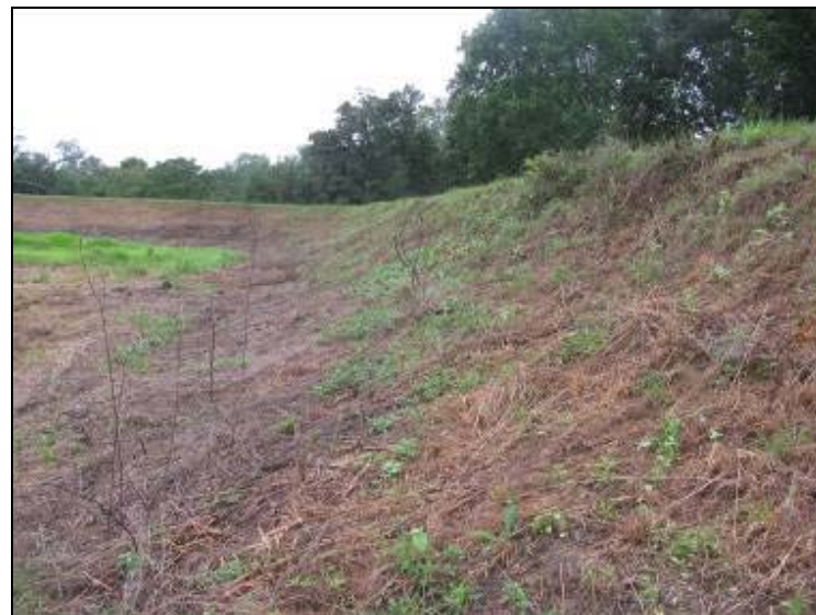
Photo 10: Ash Pond – North embankment interior slope, looking west.
