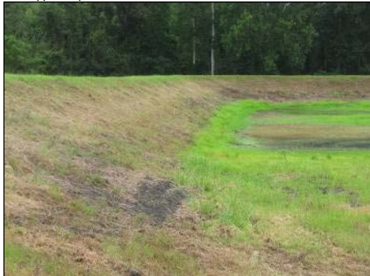
Photo 71: Ash Pond – West embankment interior slope, looking north.
