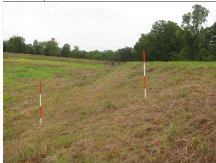
Photo 60: Ash Pond – North embankment interior slope, looking west.
