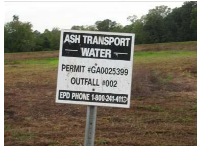
Photo 52: Ash Pond – Permit sign on southeast embankment, looking west.
