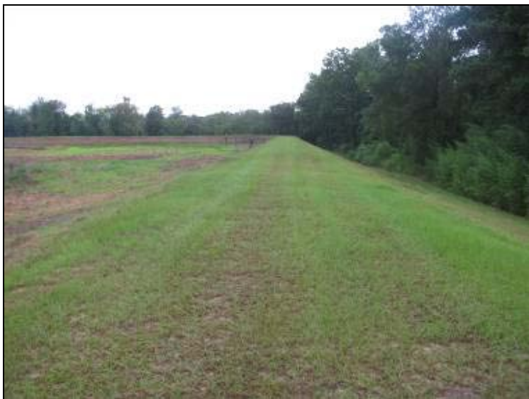
Photo 1: Ash Pond – Crest of north embankment, looking west.
