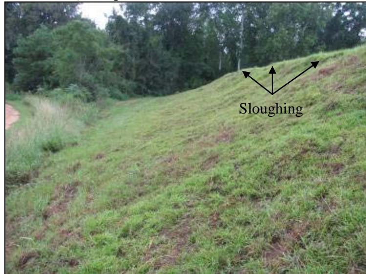
Photo 27: Ash Pond – West embankment exterior slope, looking north.
