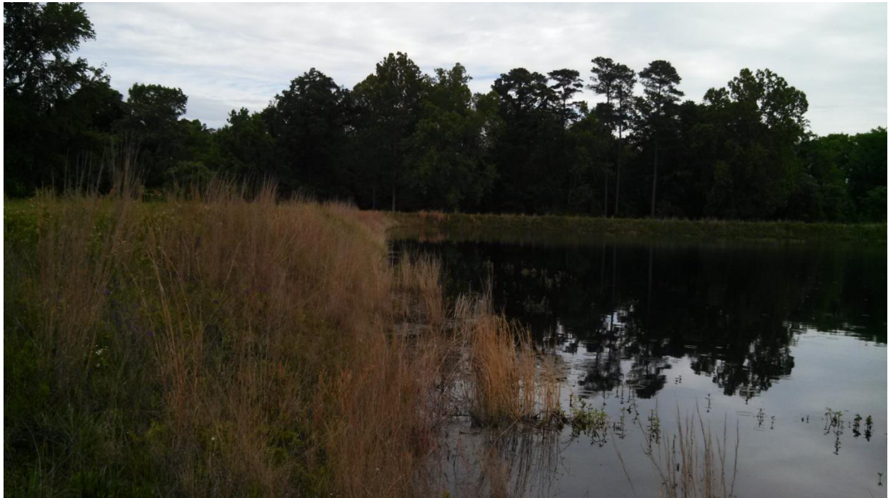
PHOTO 45 INTERIOR SLOPES OF W EMBANKMENT (LOOKING N)
