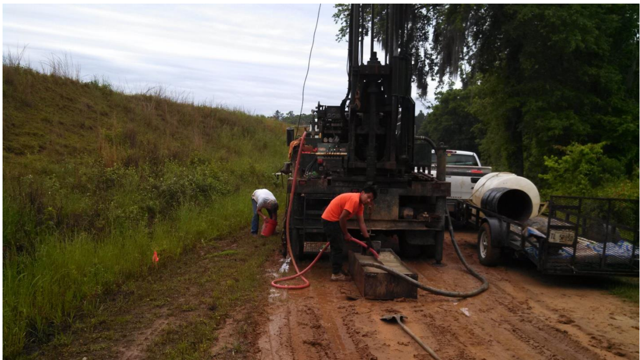
PHOTO 43 DRILLING BORING W-2
