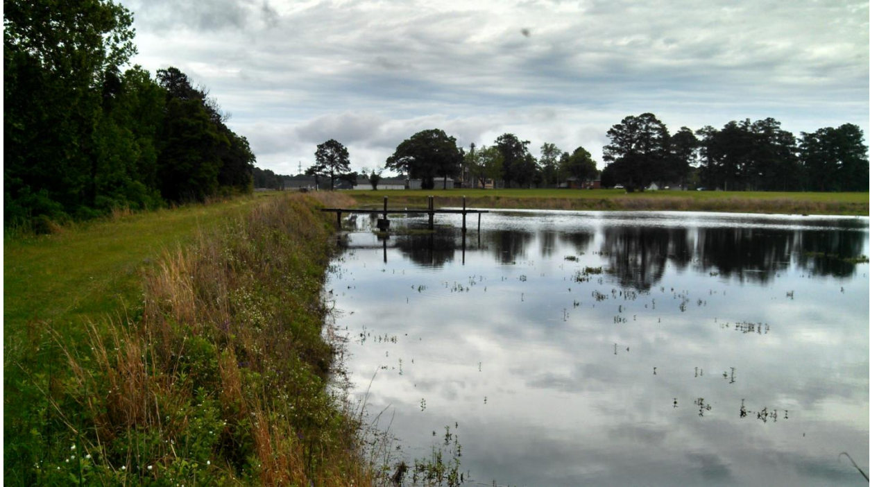
PHOTO 11 INTERIOR SLOPES OF N. EMBANKMENT FROM NW CORNER (LOOKING E)
