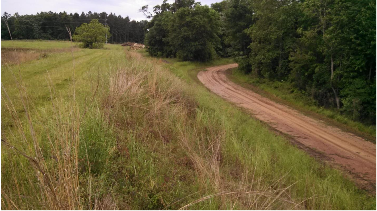
PHOTO 38 W EMBANKMENT EXTERIOR SLOPE (LOOKING S)
