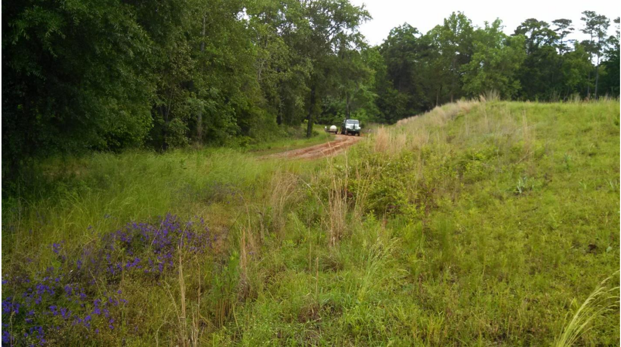
PHOTO 36 W EMBANKMENT EXTERIOR SLOPE FROM SW CORNER (LOOKING N)
