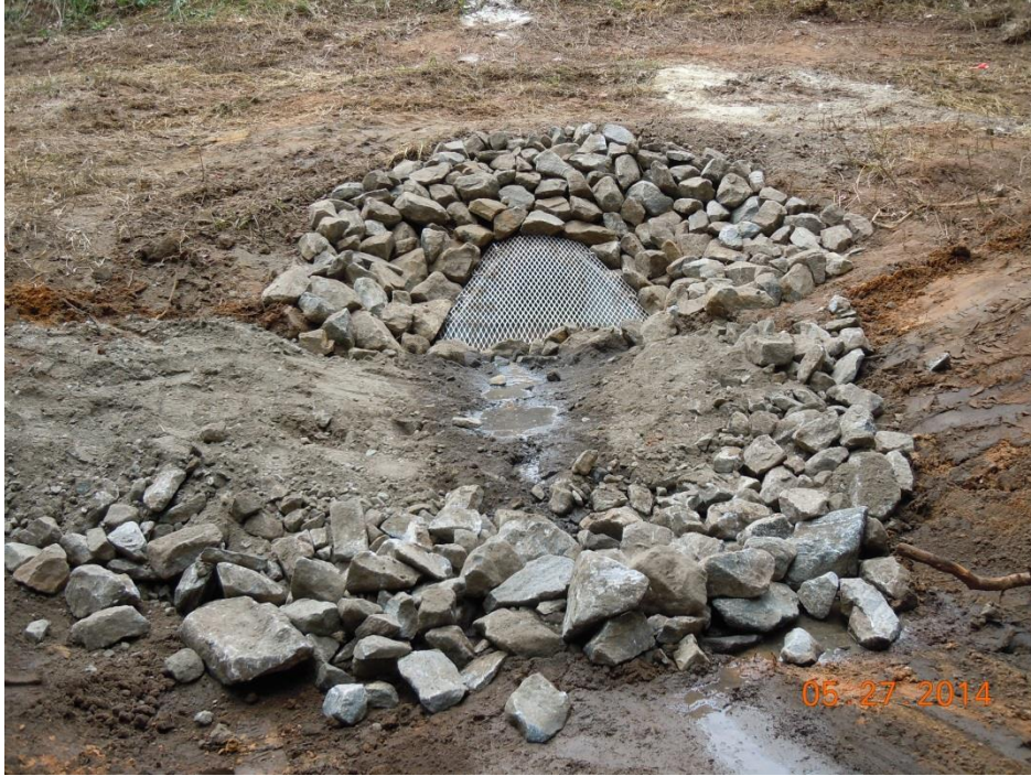
PHOTO 21 COMPLETED IMPROVEMENTS (PHOTO BY CCPC)
