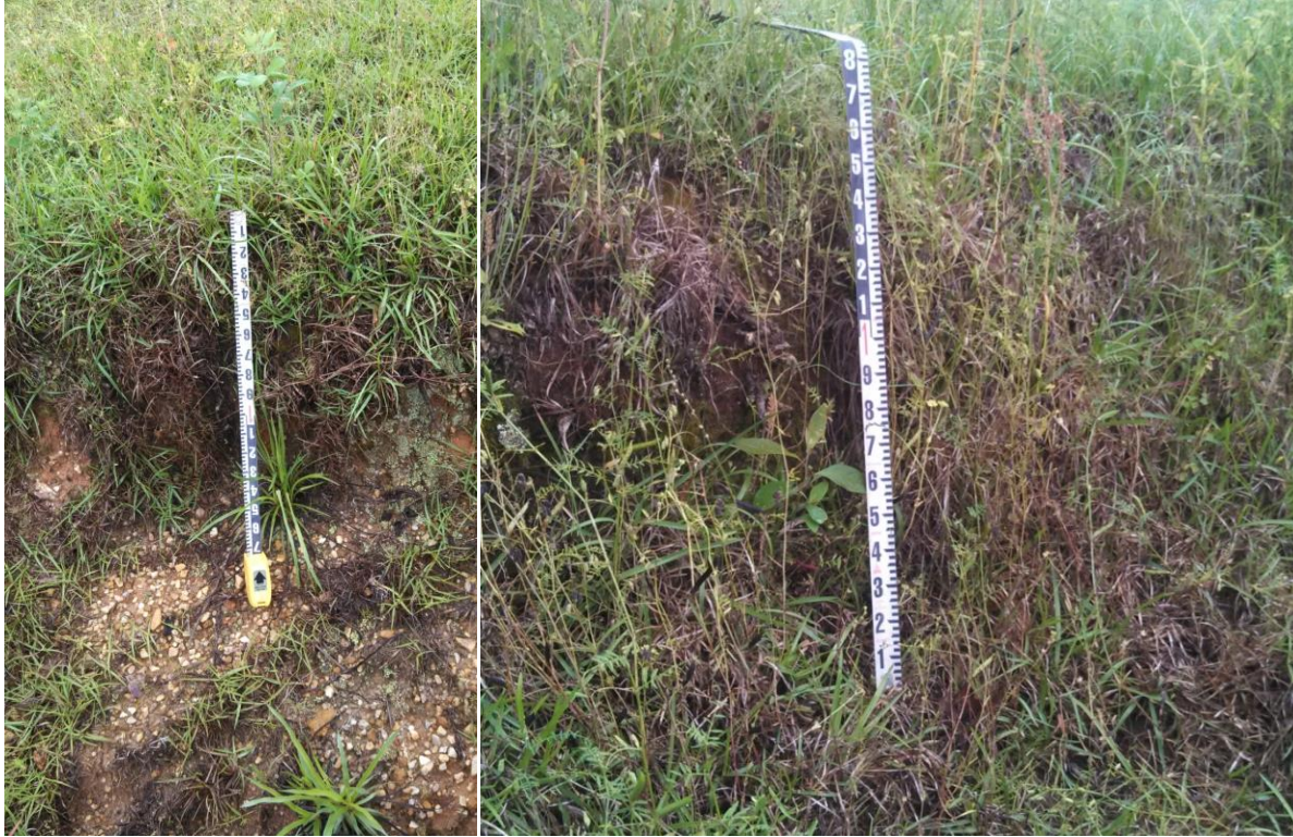
PHOTO 40 VERTICAL SURFACES AT CREST OF W EMBANKMENT
