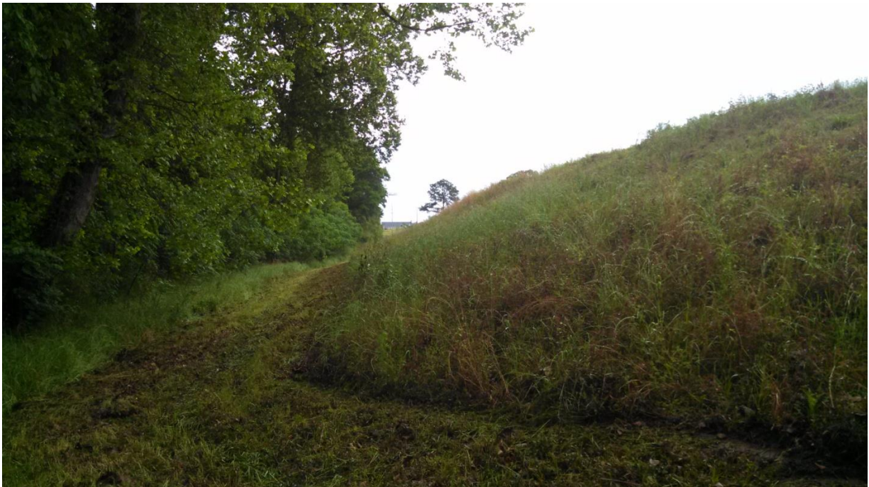
PHOTO 10 EXTERIOR SLOPES OF N. EMBANKMENT AT NW CORNER (LOOKING E)
