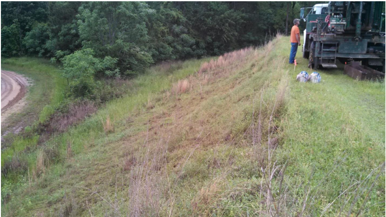
PHOTO 37 W EMBANKMENT EXTERIOR SLOPE IN HUMMOCKY/ BARE AREA (LOOKING N)
