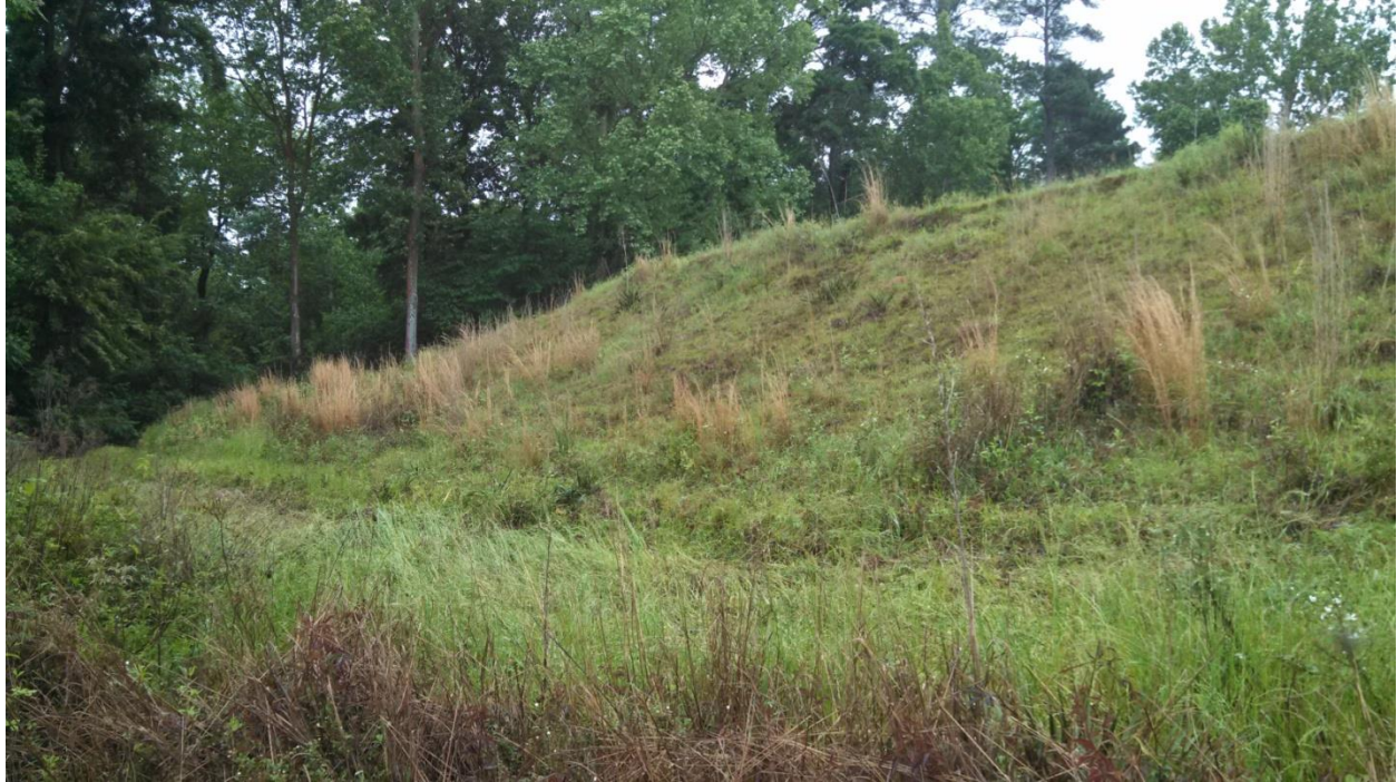
PHOTO 42 EXTERIOR SLOPES AT NW CORNER OF EMBANKMENT (LOOKING NE)
