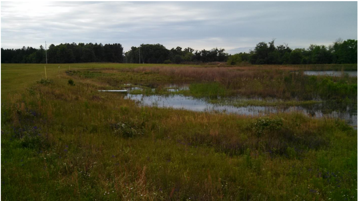
PHOTO 25 INTERIOR SLOPE OF EAST EMBANKMENT (LOOKING S)
