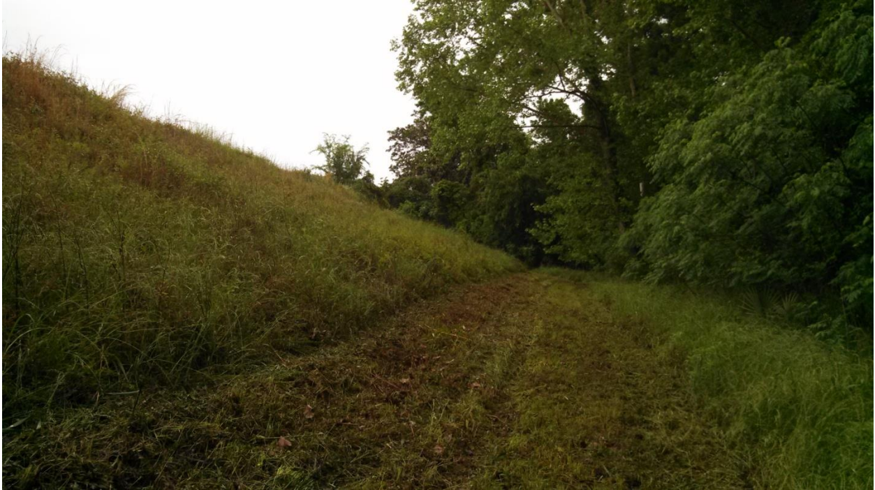
PHOTO 9 EXTERIOR SLOPES OF N. EMBANKMENT NEAR NW CORNER (LOOKING W)
