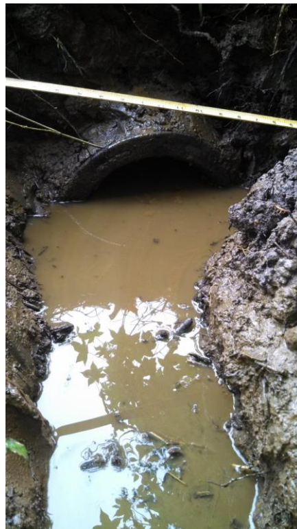
PHOTO 18 SPILLWAY DISCHARGE AFTER FLOW STOPPED
