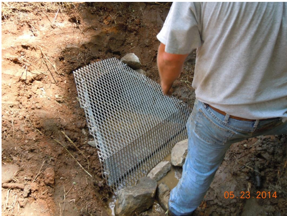
PHOTO 20 GRATE BEING INSTALLED OVER DISCHARGE (PHOTO BY CCPC)
