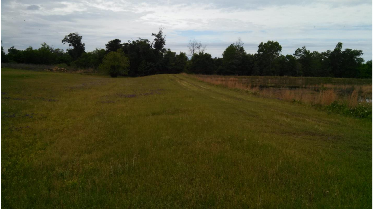
PHOTO 31 EXTERIOR SLOPES OF S EMBANKMENT FROM SE CORNER (LOOKING W)
