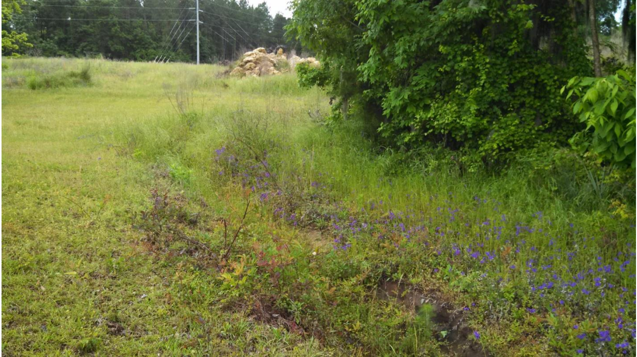
PHOTO 35 BEGINNING OF TOE DITCH AT SW CORNER OF EMBANKMENT
