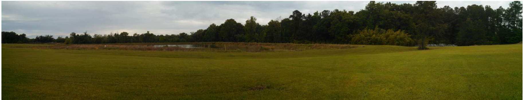
PHOTO 1 PANORAMA OF EAST EMBANKMENT (LOOKING WEST)
