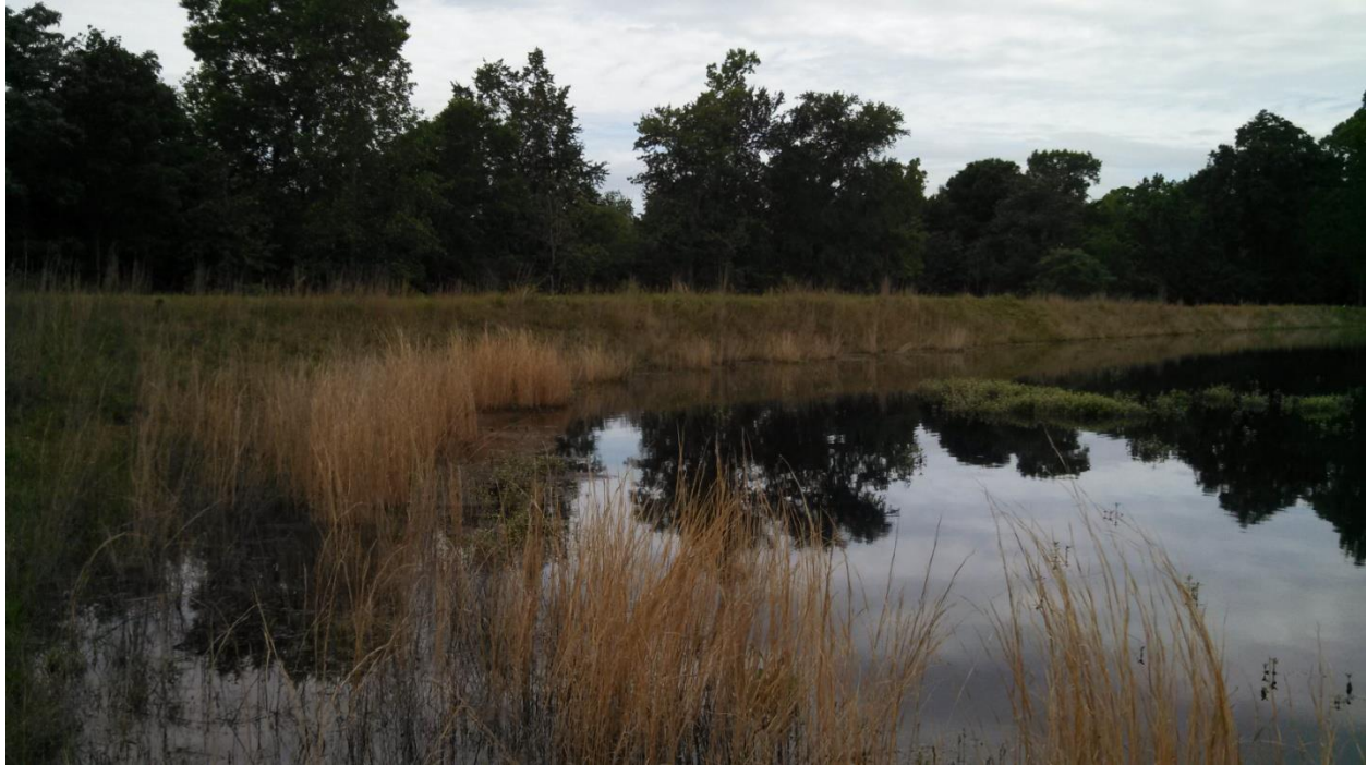
PHOTO 46 INTERIOR SLOPES OF W EMBANKMENT (LOOKING NW)
