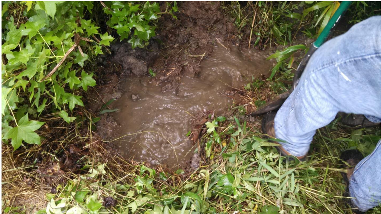
PHOTO 16 INITIAL FLOW FROM SPILLWAY DISCHARGE AFTER UNPLUGGING
