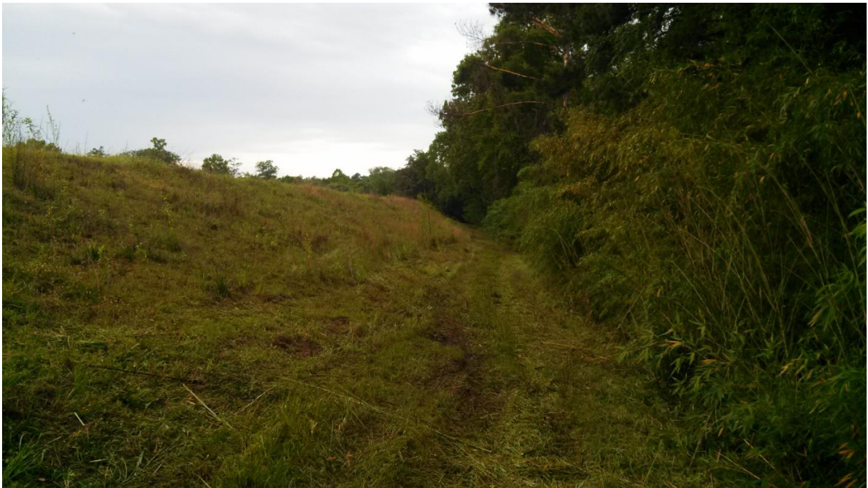
PHOTO 6 EXTERIOR SLOPES OF N. EMBANKMENT (LOOKING W FROM NE CORNER)
