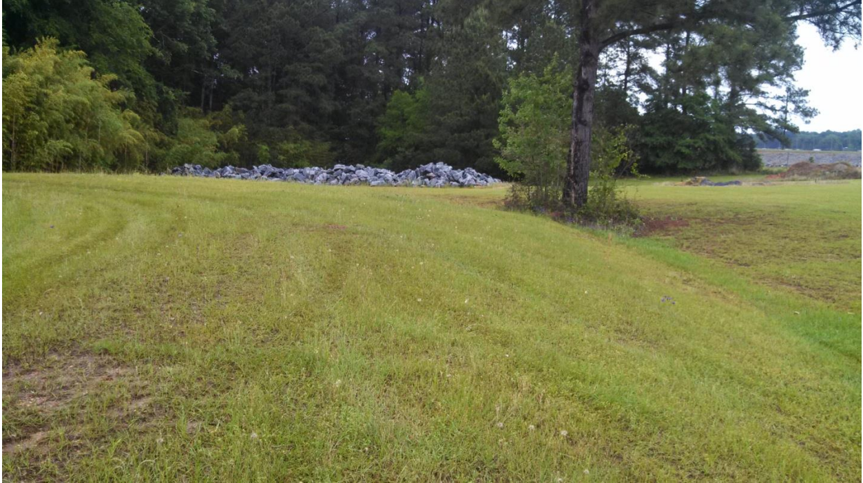
PHOTO 24 NE CORNER OF EMBANKMENTS
