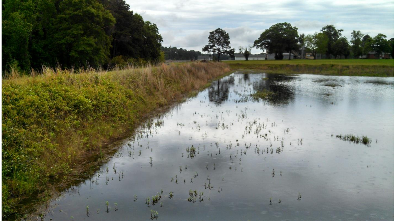
PHOTO 13 INTERIOR SLOPES OF N. EMBANKMENT FROM BOARDWALK (LOOKING E)
