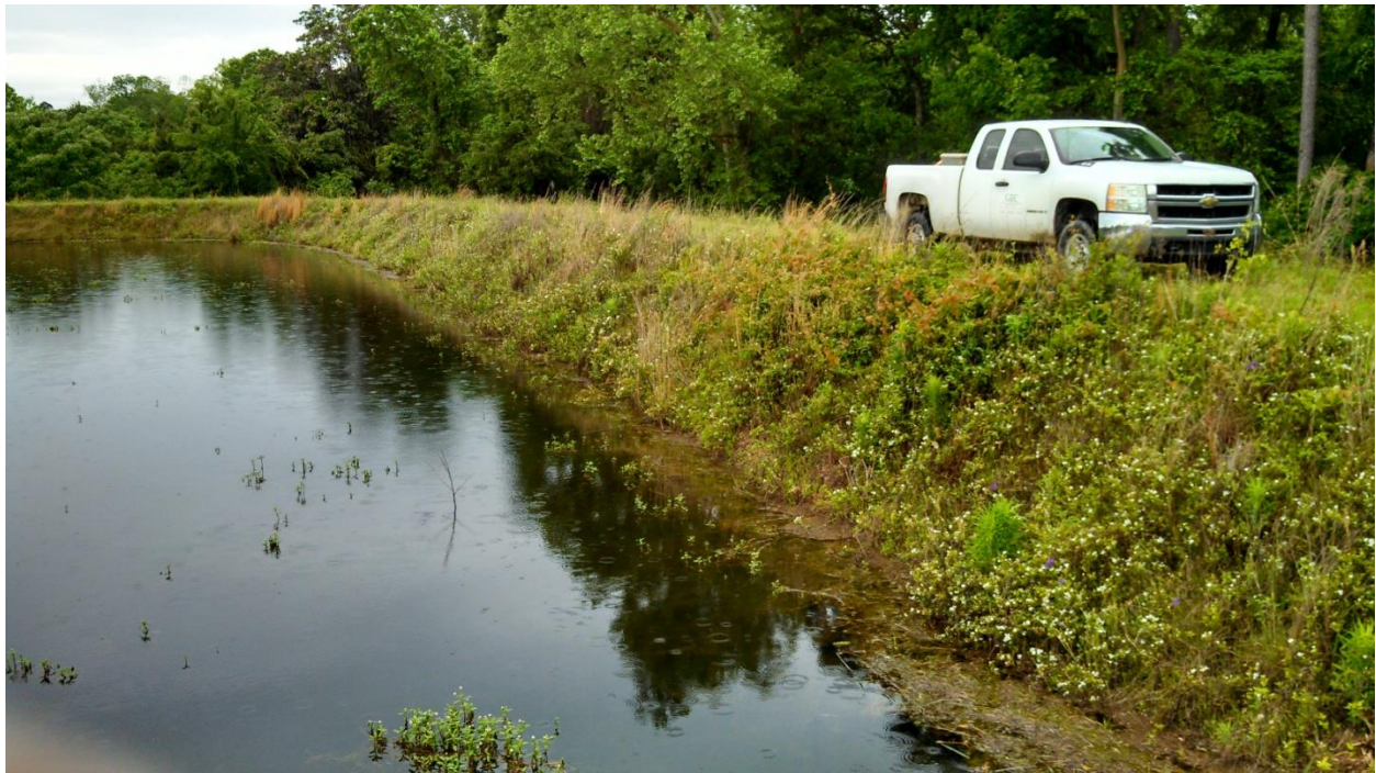
PHOTO 12 INTERIOR SLOPES OF N. EMBANKMENT FROM BOARDWALK (LOOKING W)
