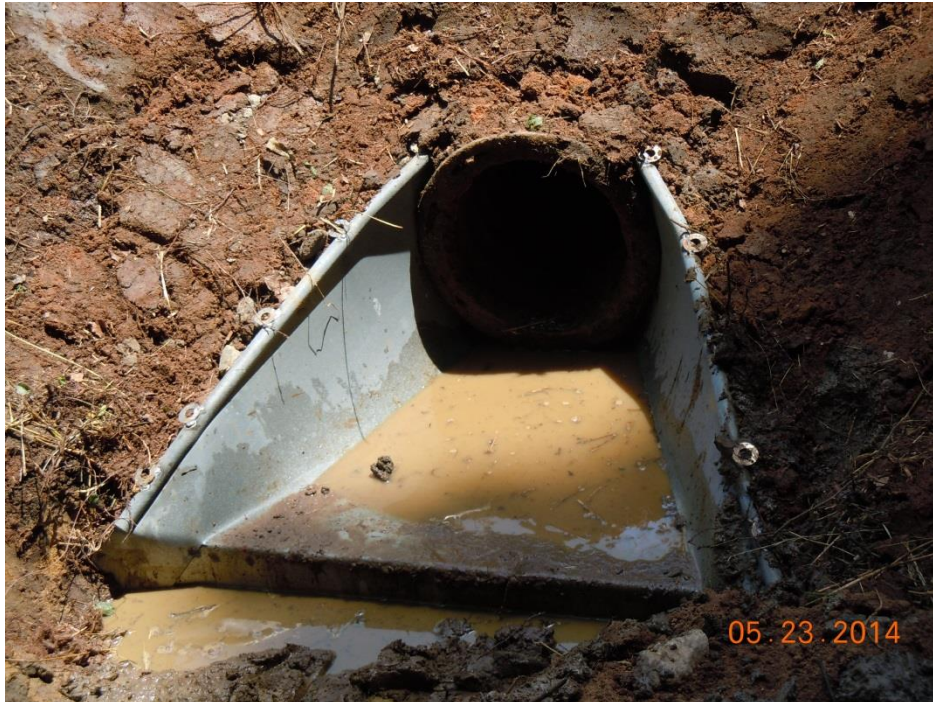
PHOTO 19 FLARED END-SECTION ADDED TO SPILLWAY DISCHARGE (PHOTO BY CCPC)
