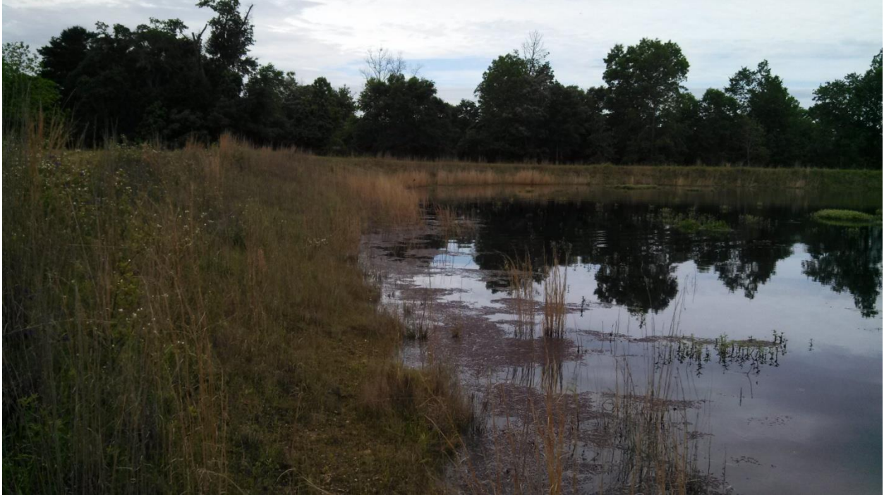
PHOTO 33 INTERIOR SLOPES OF S EMBANKMENT (LOOKING W)
