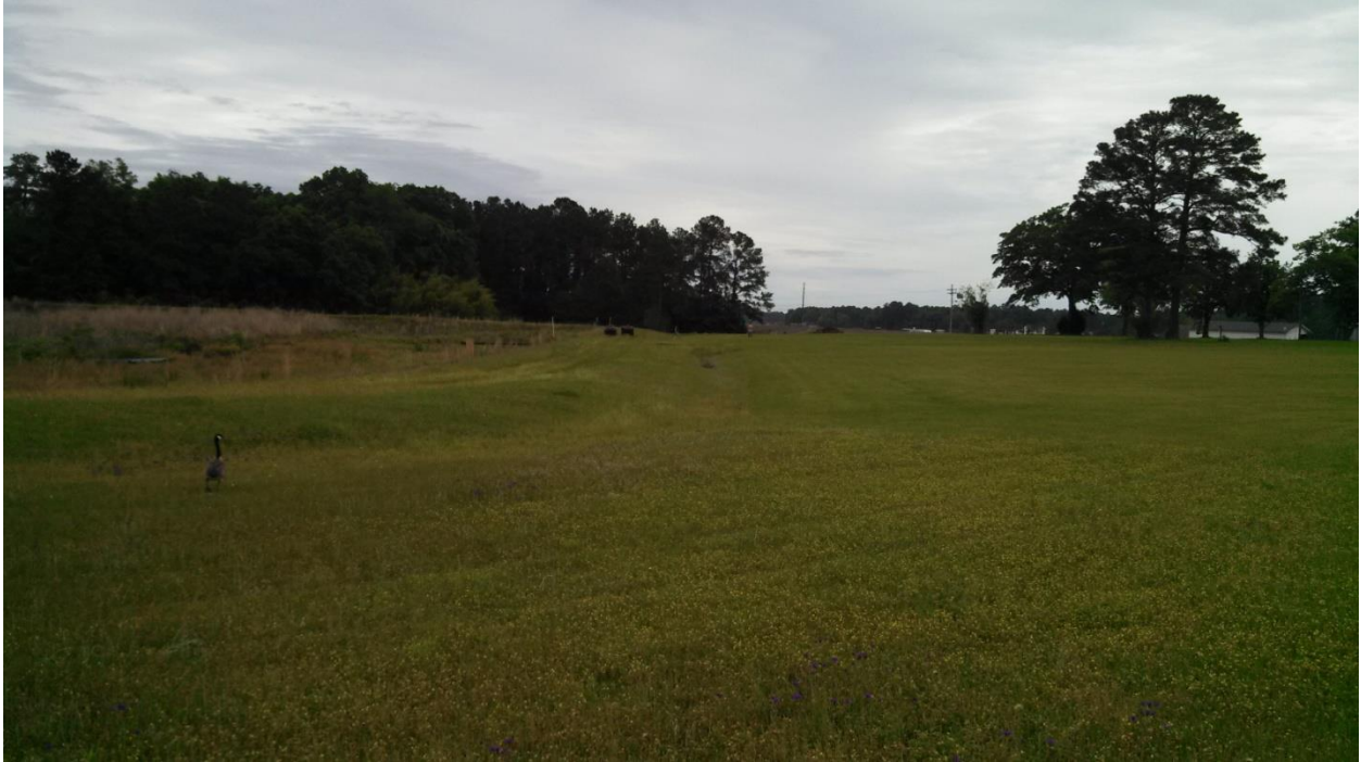
PHOTO 26 EXTERIOR SLOPE OF EAST EMBANKMENT (LOOKING N)
