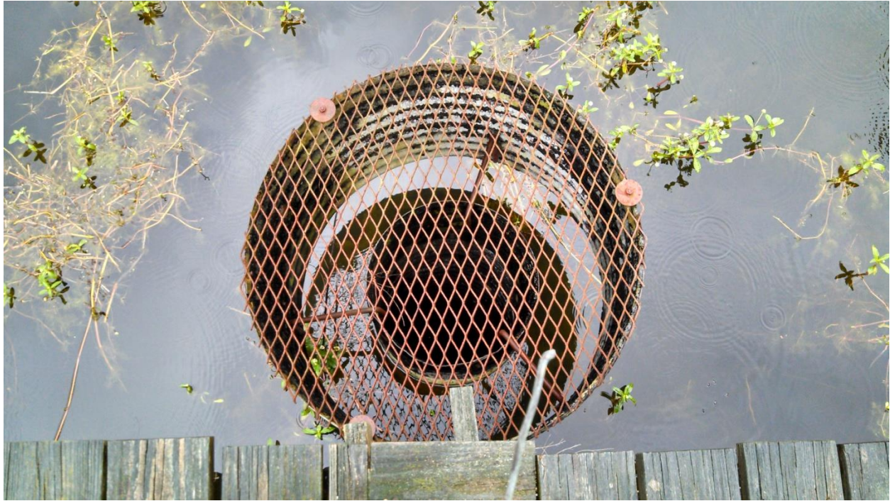
PHOTO 15 12" CMP DROP INLET AND 24" TRASH SCREEN
