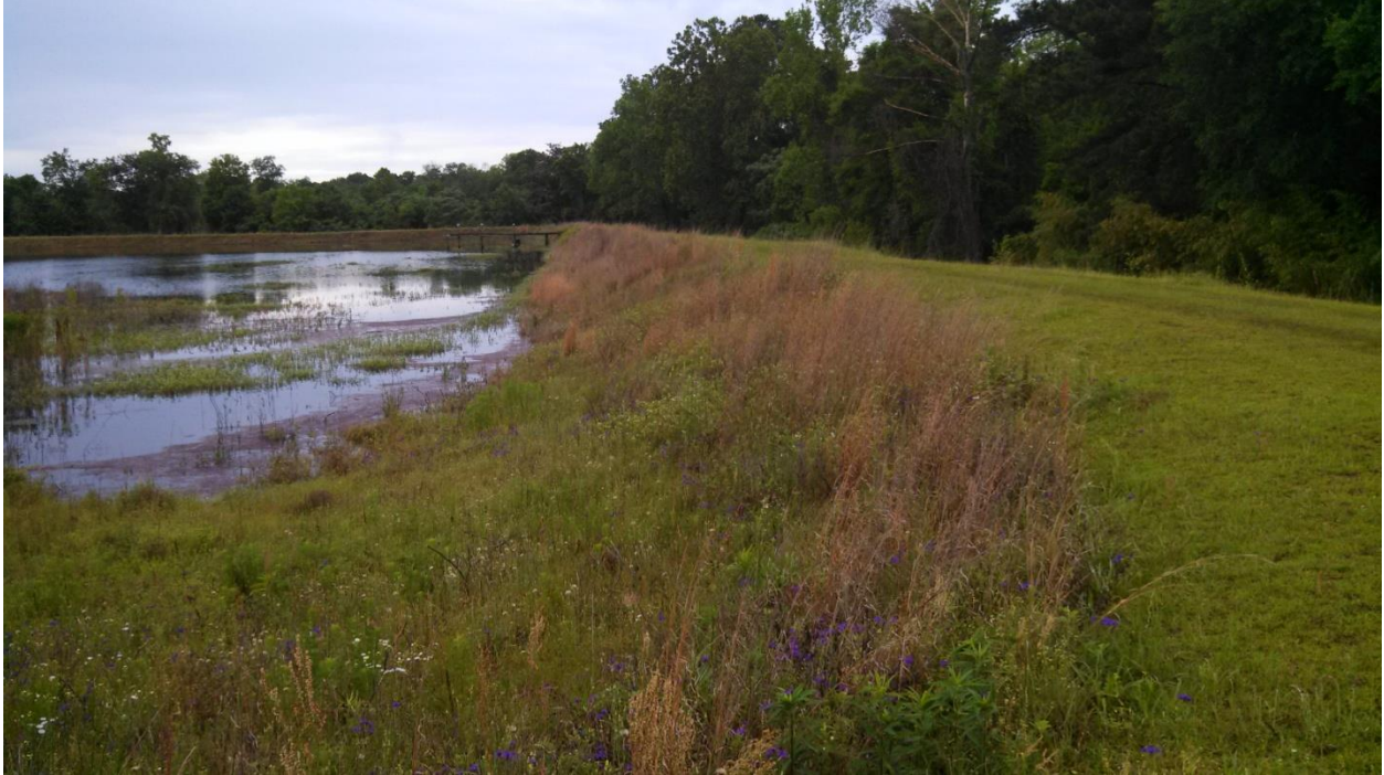
PHOTO 5 INTERIOR SLOPES OF N. EMBANKMENT (LOOKING W FROM NE CORNER)
