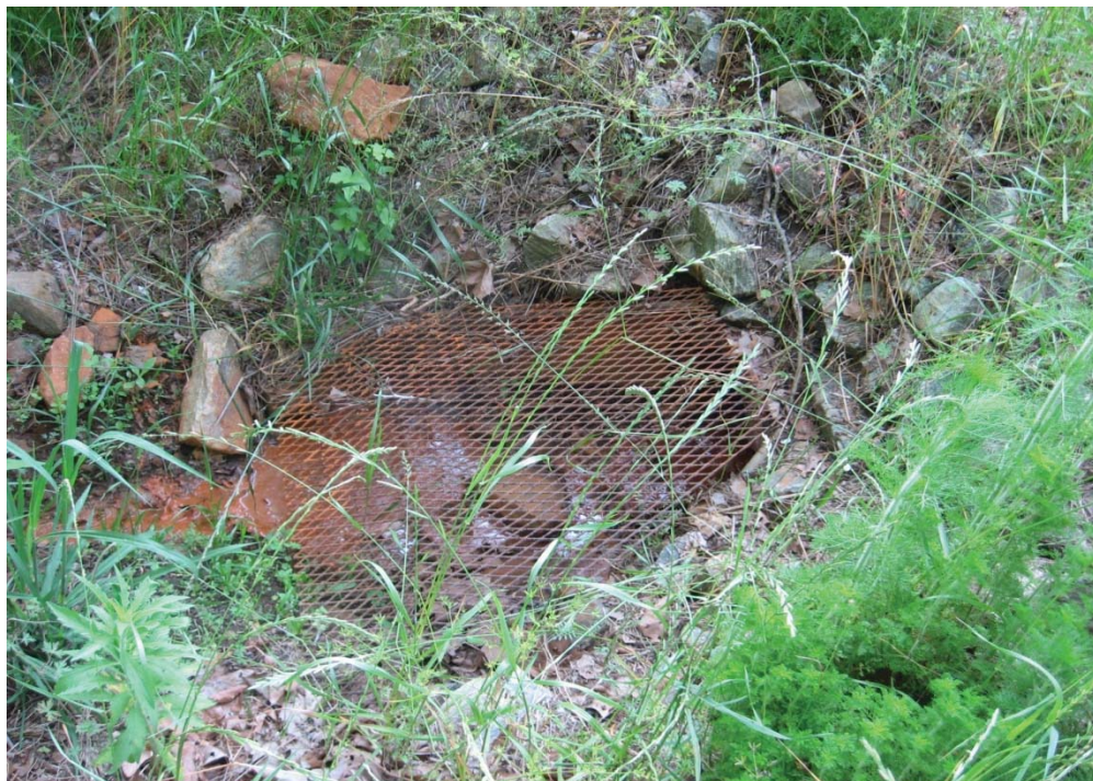
Principal Spillway Downstream Discharge Area
