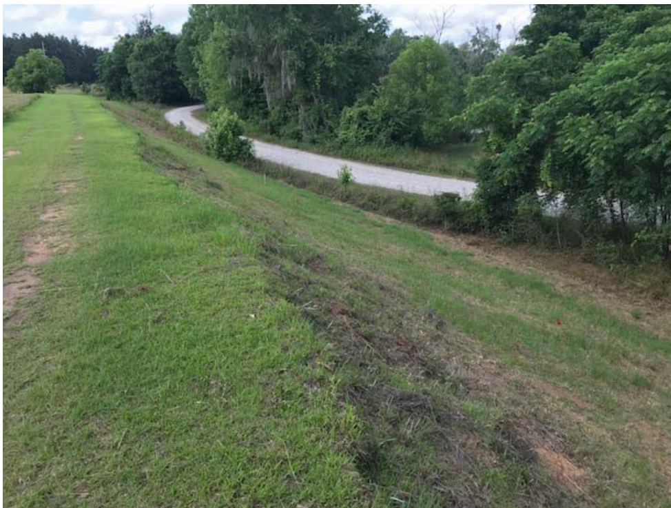
Looking South Along West Embankment After Mowing
