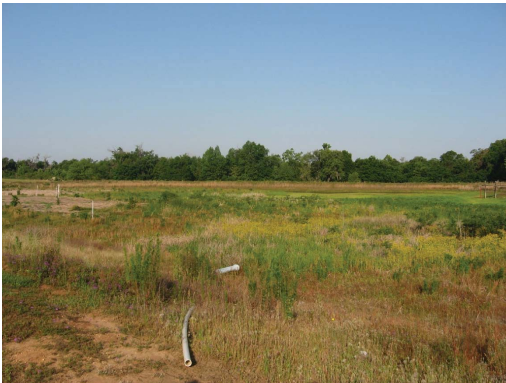
CCW Sluice Discharge at East Embankment
