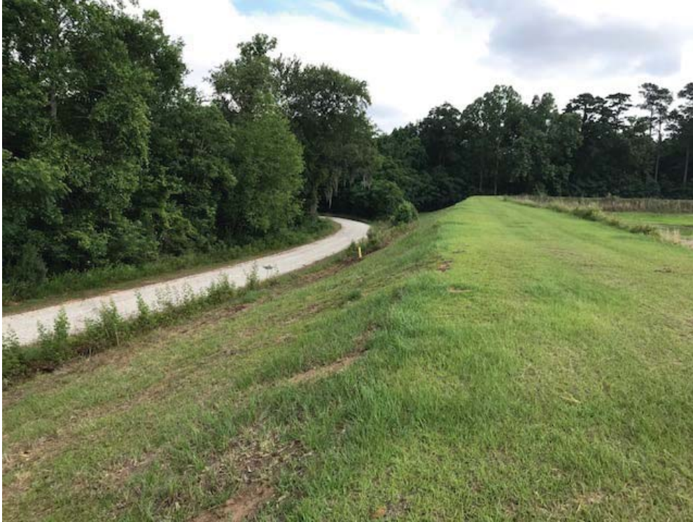
Looking North Along West Embankment After Mowing
