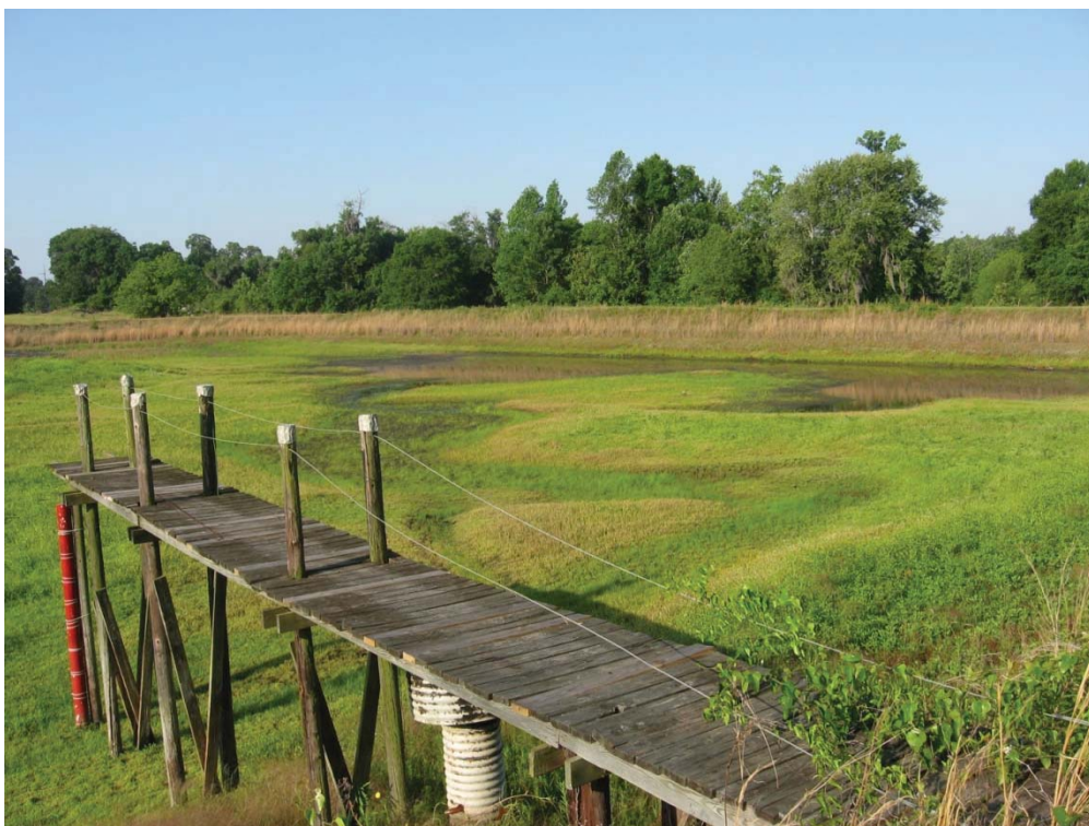
Principal Spillway Intake Riser Beneath Walkway
