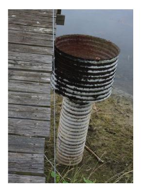
PHOTOGRAPH 9 SPILLWAY DROP INLET
